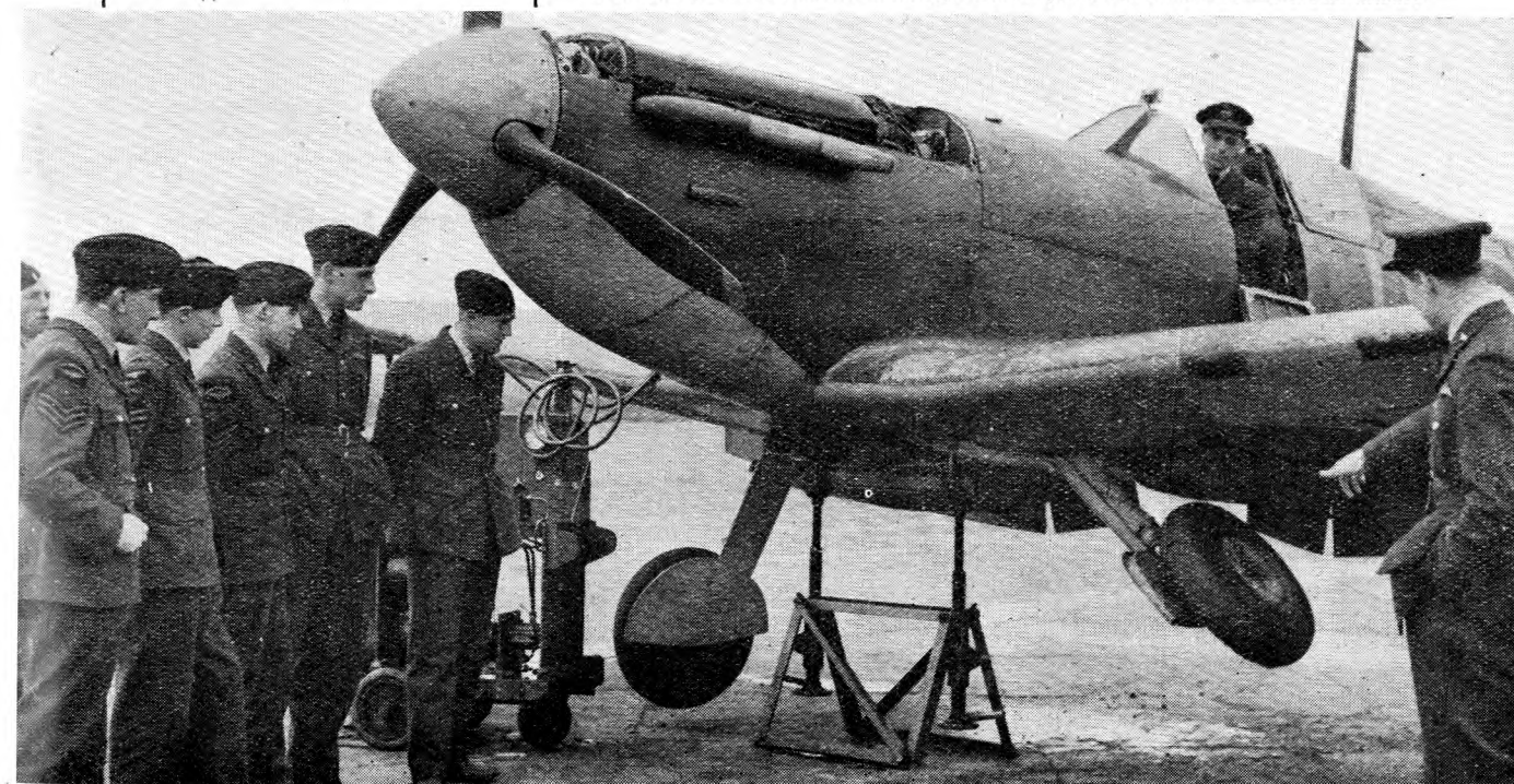
A trestle-type jack supporting a Spitfire during a demonstration of undercarriage retraction. The special bar that fits in the adjustable U pieces can be seen behind the air intake.
