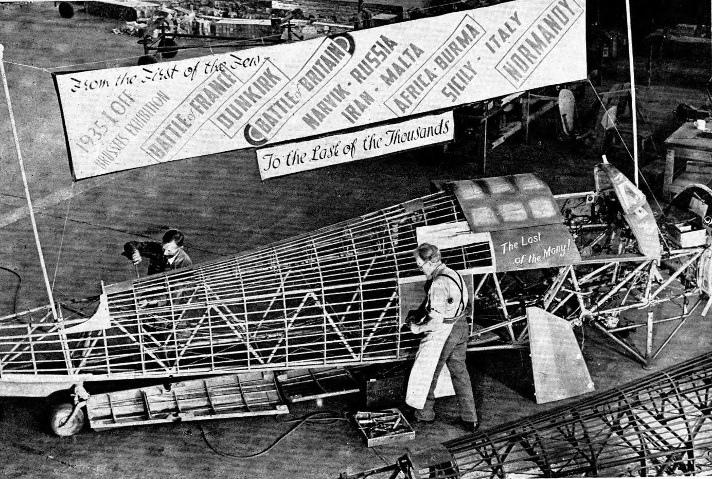
THE LAST OF THE MANY. After five years of war the Hurricane has gone out of production, though it is still in wide use. First used in the first Battle of France, the Hurricane was the most numerous fighter in the Battle of Britain, and underwent many modifications as the war developed before finally giving way to the Typhoon and the Tempest. Here the last one to be built is seen under construction and in the air.
