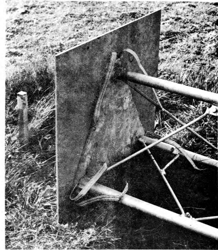
FIG. 7. FITTED BASEPLATE & EARTHING BRAIDS
