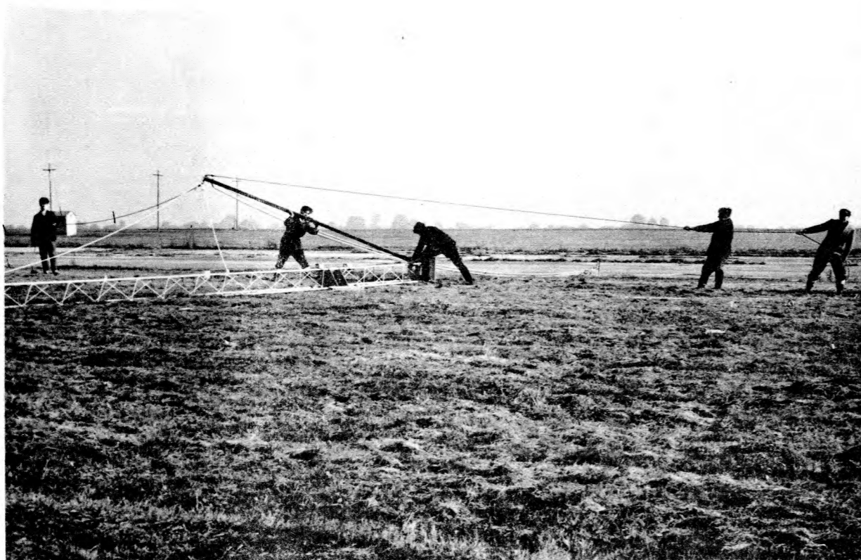
FIG. 16 . ERECTION OF DERRICK POLE
