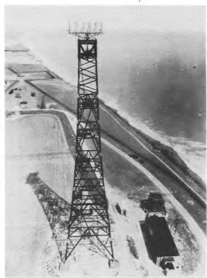
Chain Home Low Aerial, mounted on a 360 degree tower.
