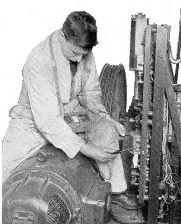
Fig. 1.—THE MEGGER CIRCUIT-TESTING OHMMETER IN USE.
