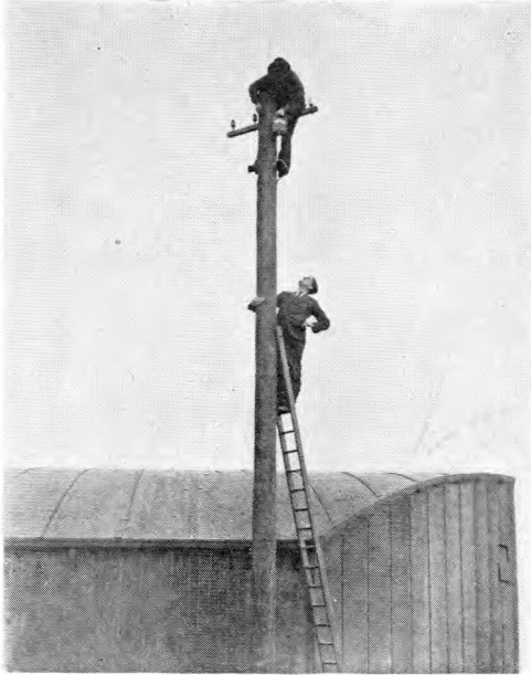
TRACING FAULTS BY TAKING AVOMETER READINGS.
