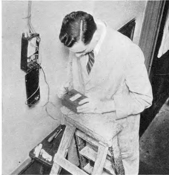
TEST TO EARTH ON A HOUSE INSTALLATION.
