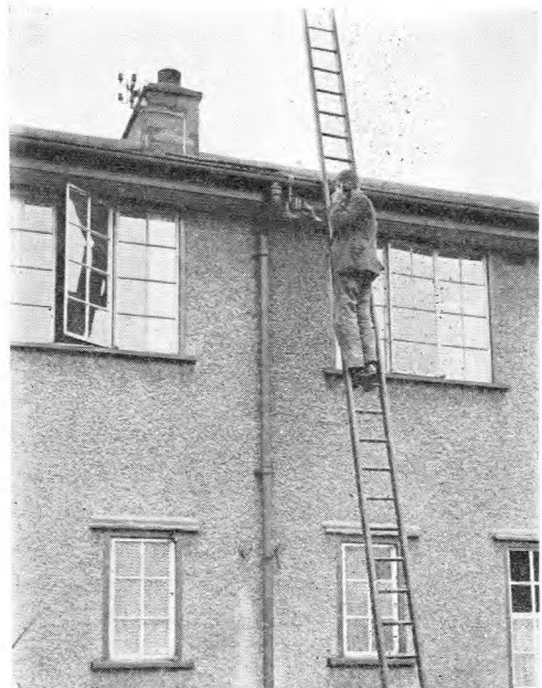
TESTING WITH TELEPHONES ON A THREE-WAY TEST BOX.
