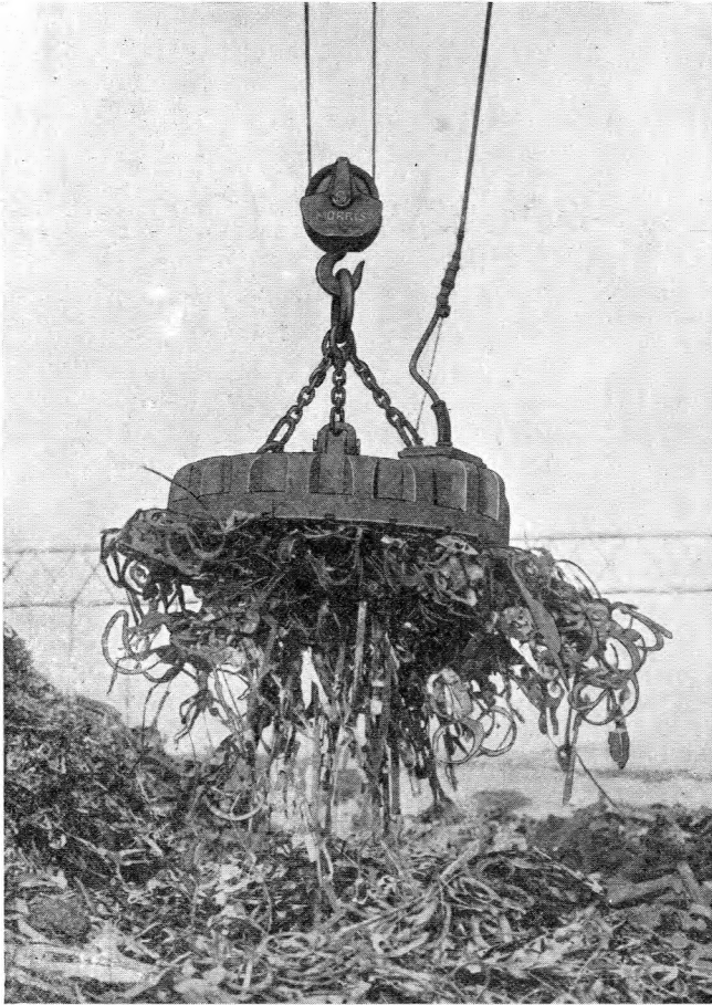
CIRCULAR MAGNET LIFTING LIGHT SCRAP AND TURNINGS.
