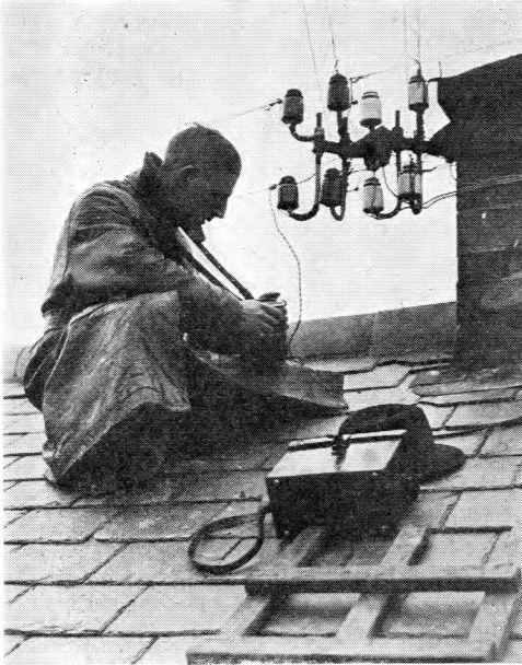
TESTING LINES TO EARTH WITH A MEGGER INSULATION TESTER.
