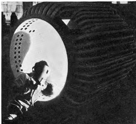
METALLIC ARC-WELDING IN PROGRESS AT THE B.T.H. WORKS, RUGBY.
