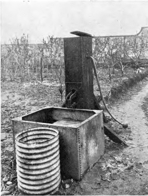
THE PUMP BEFORE CONVERSION TO ELECTRIC OPERATION. (B.T.H.)
