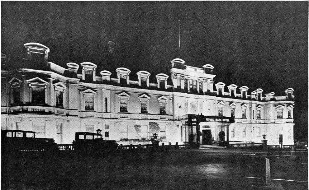
SHOWING THE USE OF MAZDA MERCRA LAMPS FOR FLOODLIGHTING THE ROYAL BATH HOTEL, BOURNEMOUTH.
