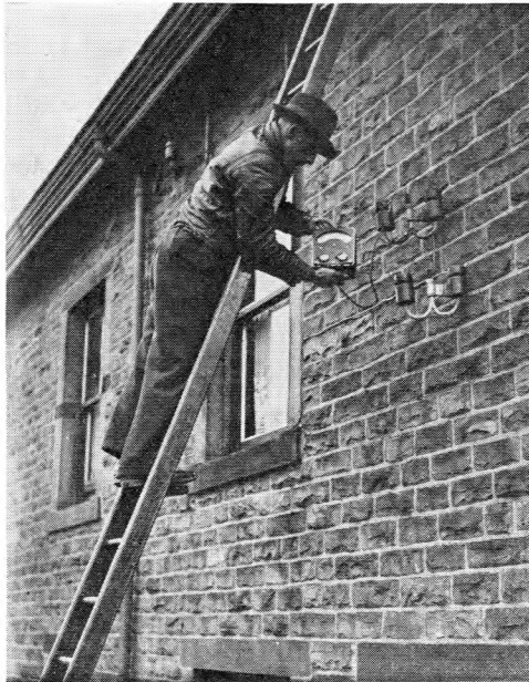
MEASURING RESISTANCE TO EARTH.
