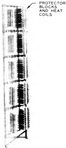
FIGURE 822. Protected Main Distributing Frame (Wall Mounted) (Western Electric Co.)
