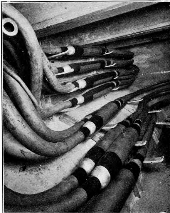
FIG. 5.—COMPLETED JOINTS IN MANHOLE OUTSIDE BRETENHAM HOUSE.
