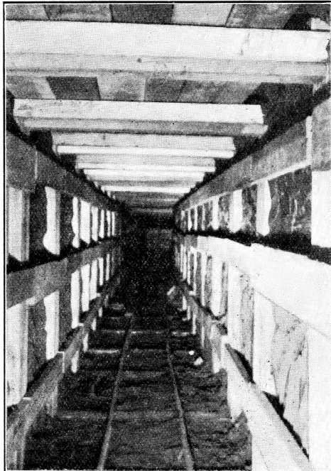
FIG. 1.—HEADING FOR 99-WAY DUCT ROUTE.
