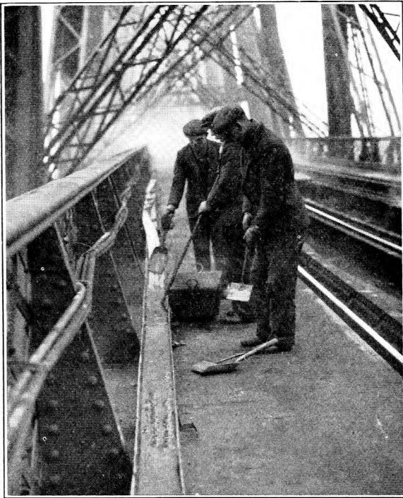
FIG. 4.—FILLING THE TROUGH WITH COMPOUND.
