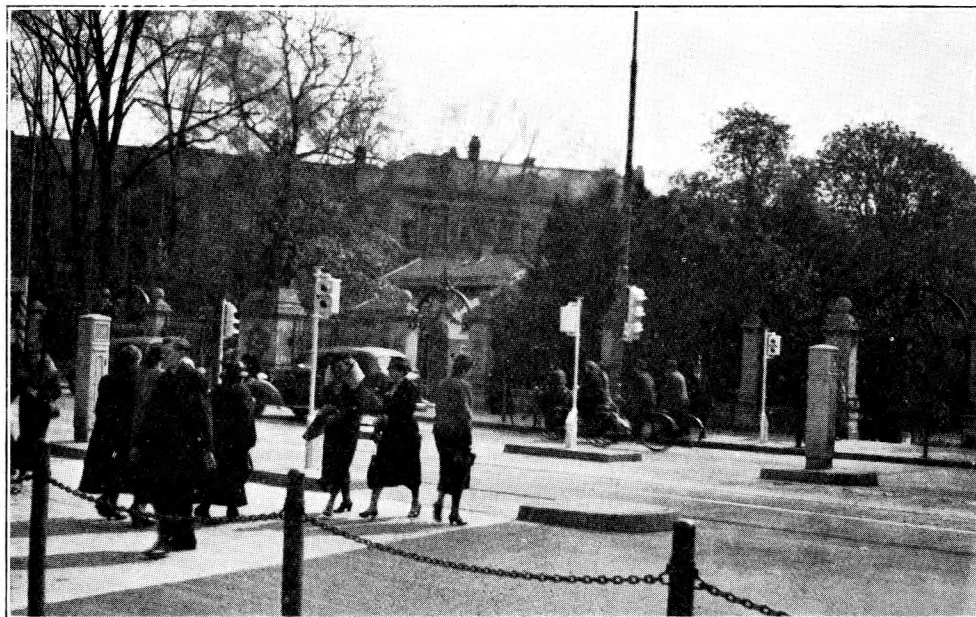
FIG. 14.—PEDESTRIAN CROSSING WITH SIGNAL LIGHTS.
