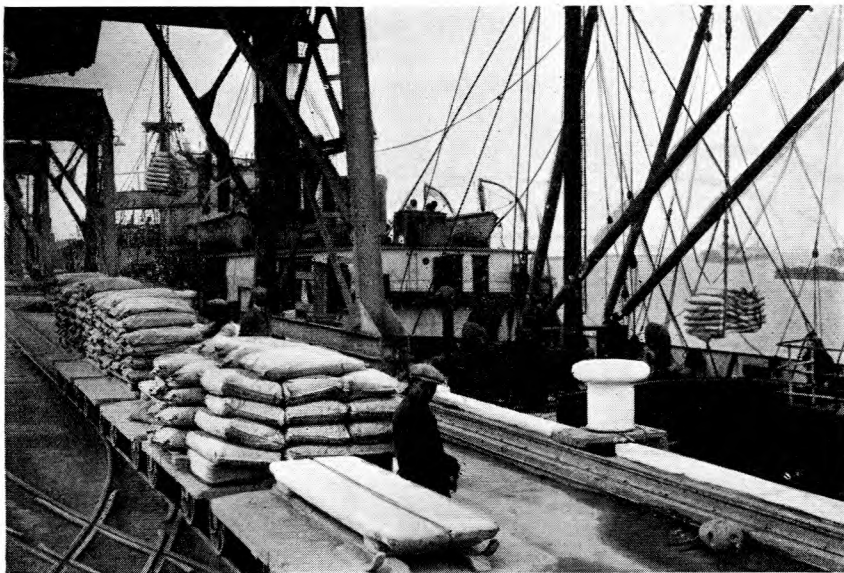
FIG. 9.—LOADING CEMENT IN PAPER BAGS.
