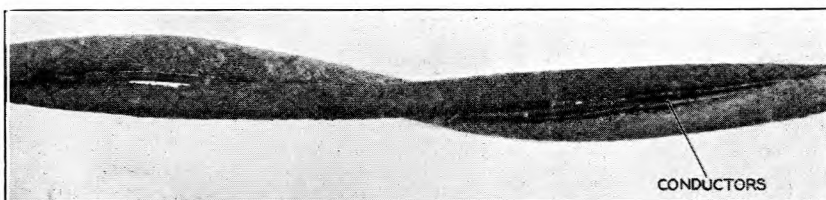
FIG. 5.—INSULATED WIRES DAMAGED BY LIGHTNING.
