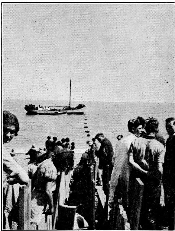
FIG. 1.—LAYING THE SHORE END AT ALDEBURGH.
