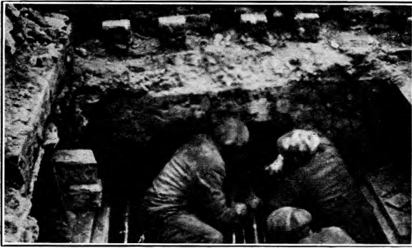
FIG. 1.—LAYING THE LAST PIPE.
