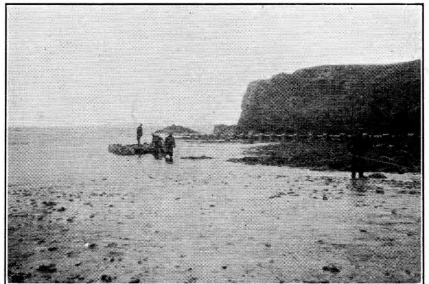
FIG. 2.—LANDING THE CABLE FROM THE RAFT.
