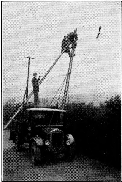
FIG. 10.—DERRICK USED TO ERECT AERIAL CABLE.
