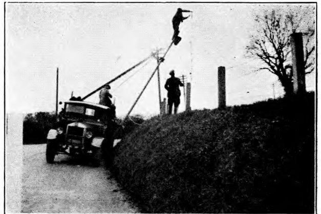
FIG. 6.—DERRICK USED WITH MAXIMUM OVERHANG.
