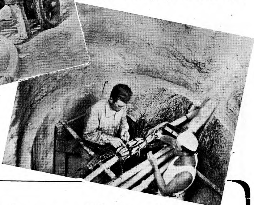
Jointing operations in progress.
