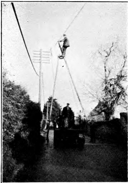
FIG. 7.—DERRICK USED IN VERTICAL POSITION.
