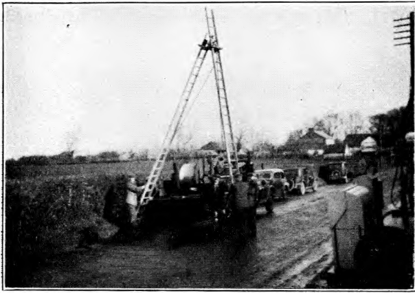
FIG. 4.—ERECTION OF DERRICK.
