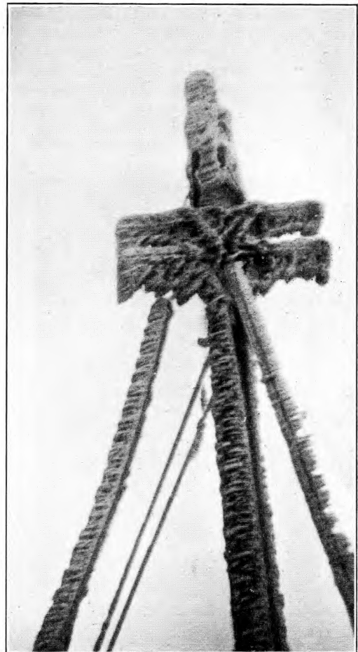
FIG. 4.—POLE HEAD ENCASED IN ICE.
