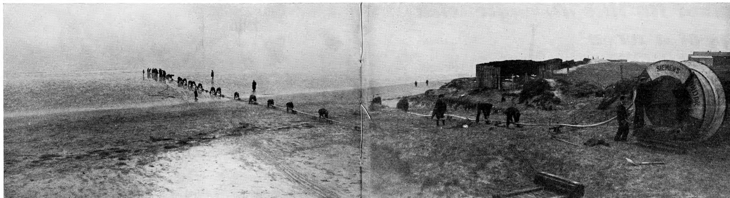
LAYING SUBMARINE TELEPHONE CABLE ACROSS AN ESTUARY
