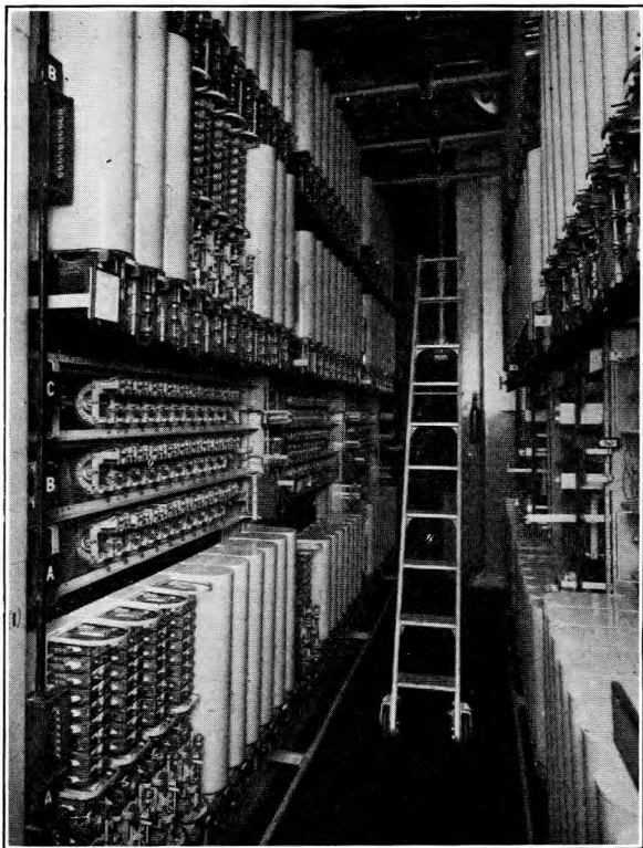
FIG. 5.—TRUNK 1ST CODE SELECTORS.
