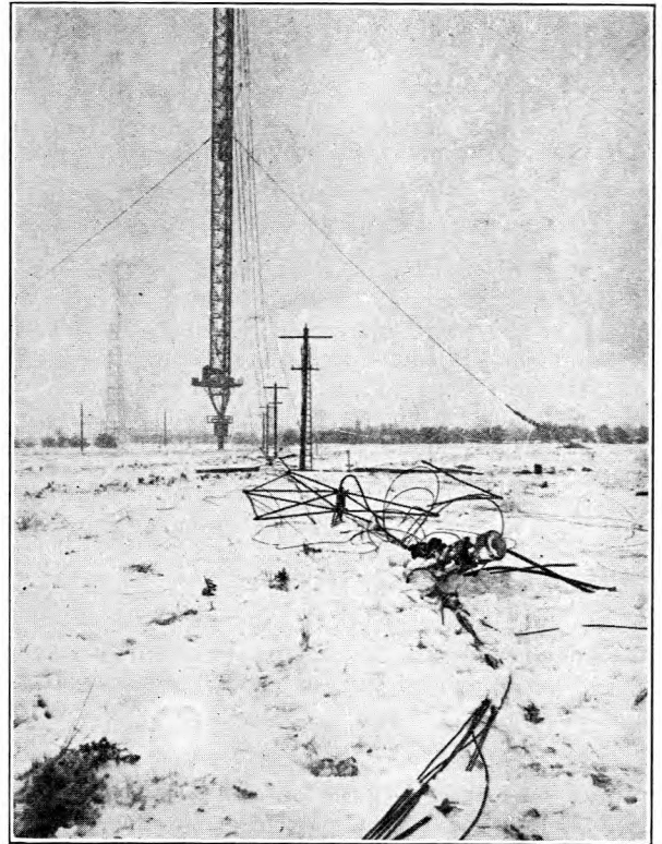
FIG. 4.—GENERAL VIEW OF FALLEN AERIAL.
