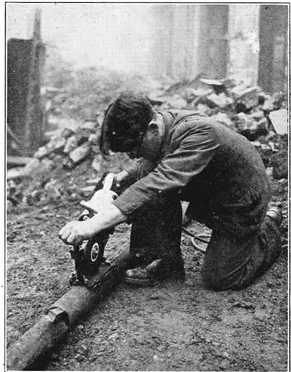
FIG. 2.—"SKILSAW" CUTTING STEEL PIPE.
