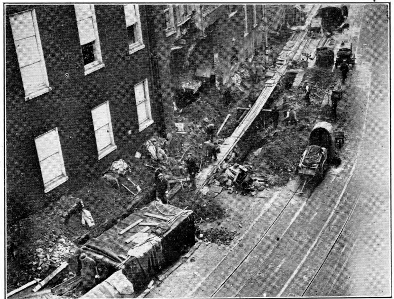
FIG. 6. BRIDGE CARRYING INTERRUPTION CABLE OVER BOMB CRATER.
