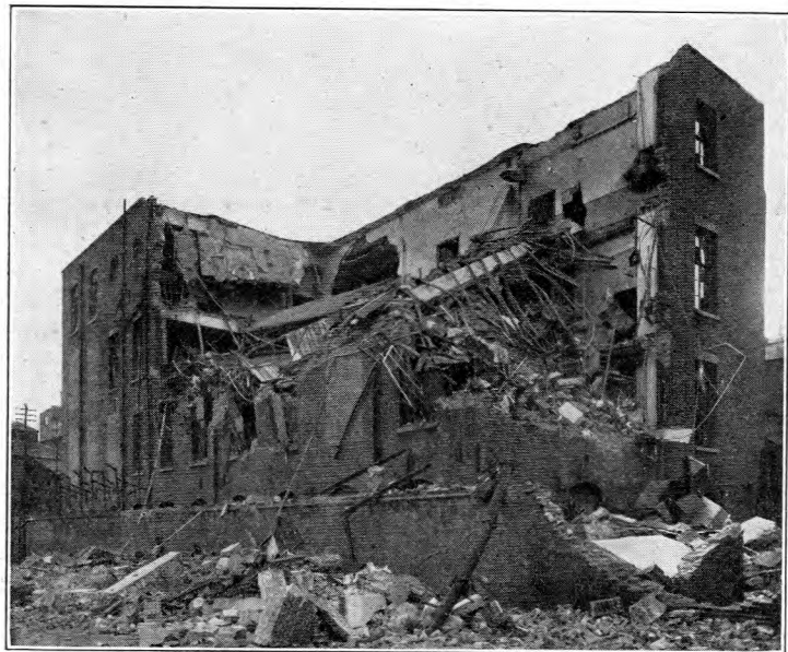
FIG. 1.—COMPLETE DESTRUCTION OF A LONDON TELEPHONE EXCHANGE BUILDING.
