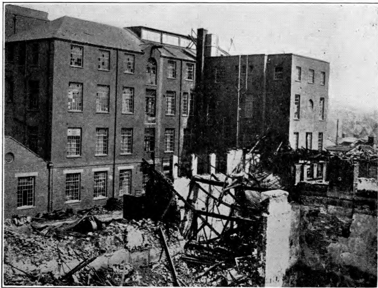
FIG. 4.—A LARGE PROVINCIAL EXCHANGE BUILDING SAVED FROM DESTRUCTION BY FIRE.
