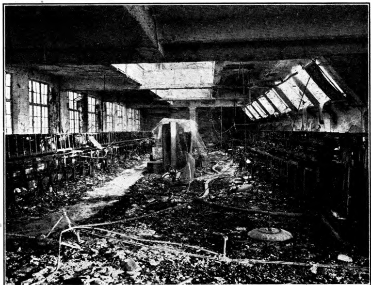
FIG. 3.—AUTO-MANUAL SWITCH ROOM. SIXTH FLOOR.
