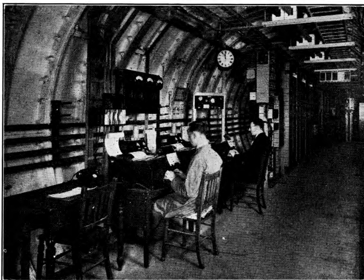
FIG. 6.—V.F. TELEGRAPH EQUIPMENT IN DEEP-LEVEL PROTECTION.
