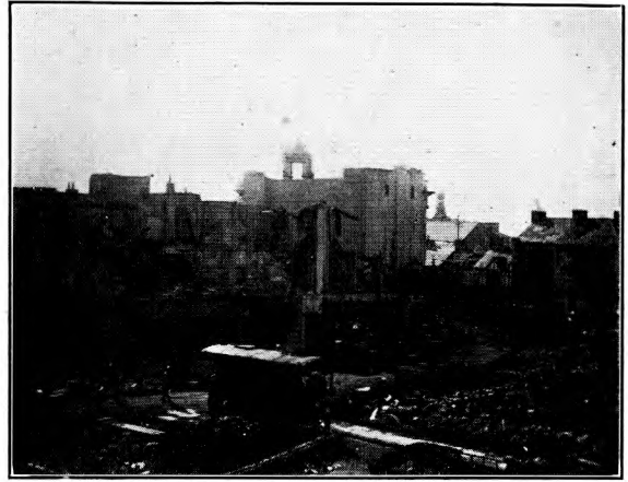
FIG. 3.—VIEW FROM TELEPHONE HOUSE, SWANSEA.
