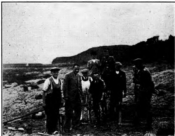
FIG. 2.—STATES TELEPHONE DEPARTMENT JOINTER WORKING UNDER ESCORT ON SUBMARINE CABLE AT FLIQUET.
