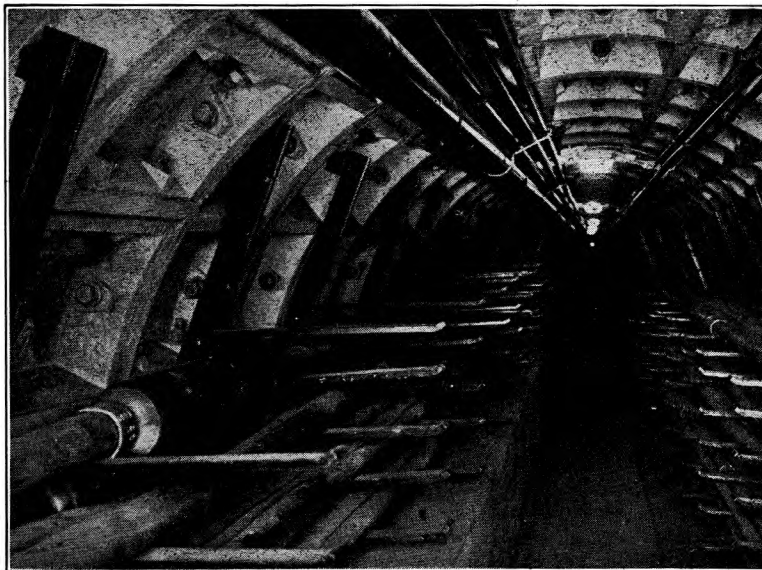
FIG. 4.—CABLES IN TUNNEL.
