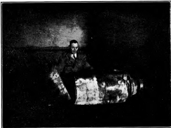
FIG. 2.—BOMB IN TELEPHONE HOUSE, SWANSEA.
