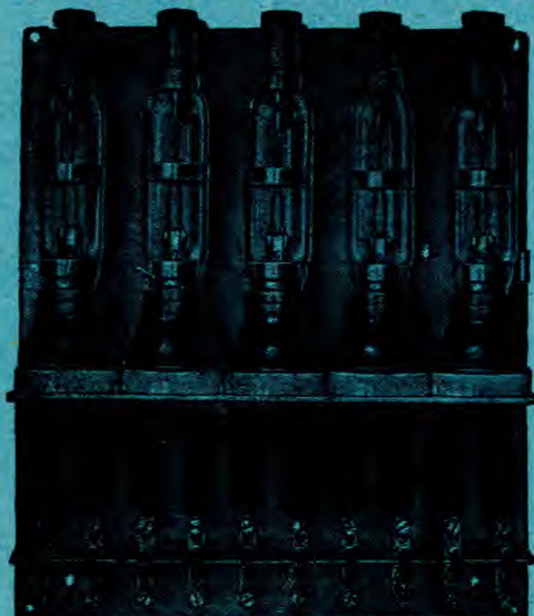
5-circuit panel for overhead lines incorporating choke coils, spark gaps, etc.
