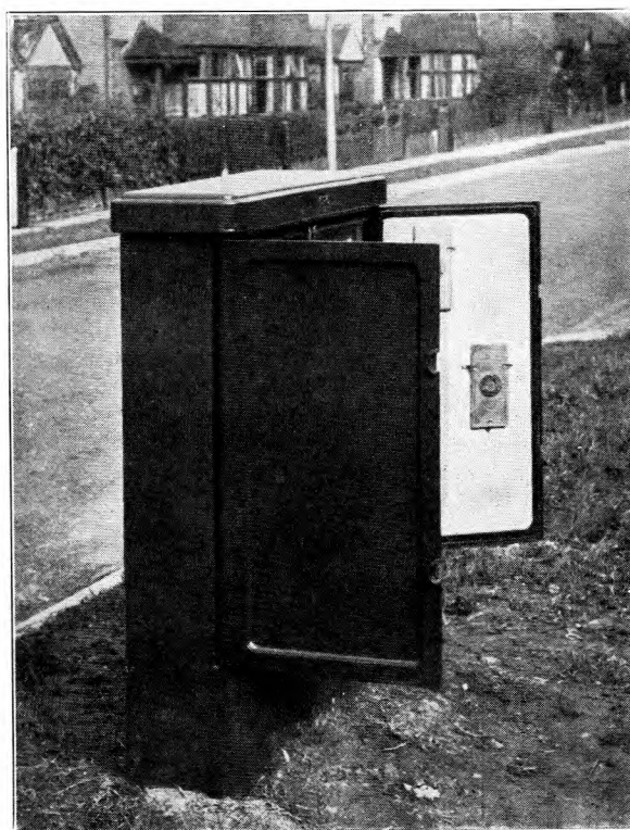
FIG. 3.—CROSS-CONNECTION CABINET.
