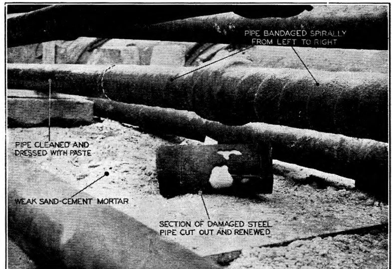
FIG. 4.—P.O. PIPE UNDER TREATMENT.
