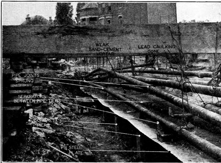
FIG. 5.—RECONDITIONING OF PIPES AT ADVANCED STAGE.
