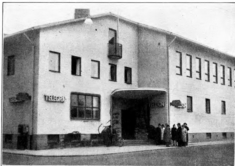
FIG. 2.—TELEGRAPH AND TELEPHONE BUILDING IN KRISTIANSTAD.
