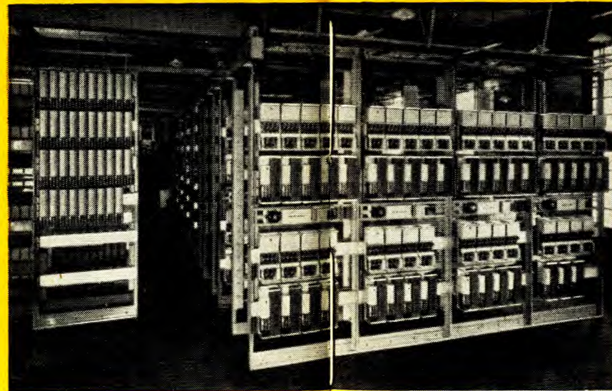
STROWGER Director and Selector Racks in operation at Johannesburg Central Exchange
