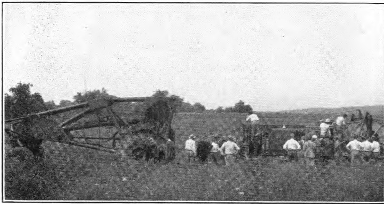
FIG. 2.—LAYING A COAXIAL CABLE BY GIANT PLOUGH.
