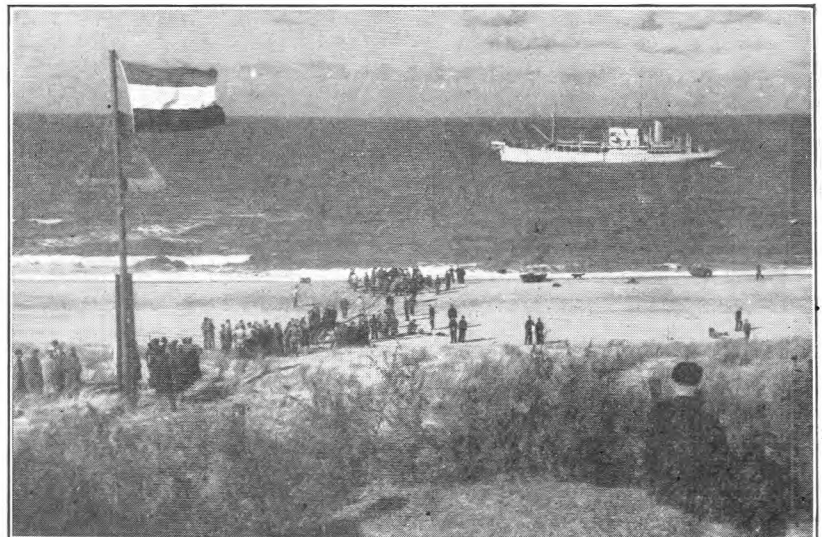
FIG. 4.—H.M.T.S. Alert LAYING SHORE END AT DOMBURG.
