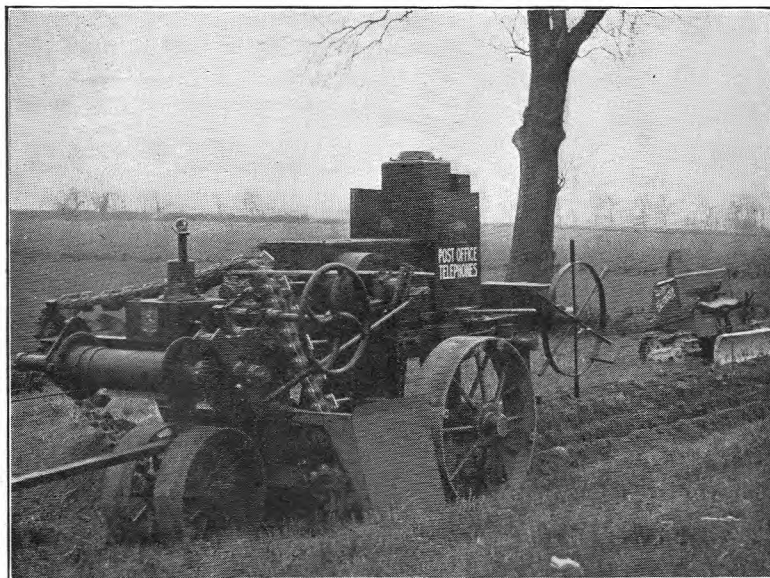
FIG. 1.—AVELING-BARFORD TRENCH-CUTTING MACHINE.
