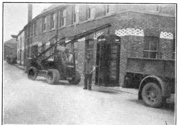
MOBILE CRANE IN USE FOR PLACING KIOSK.
