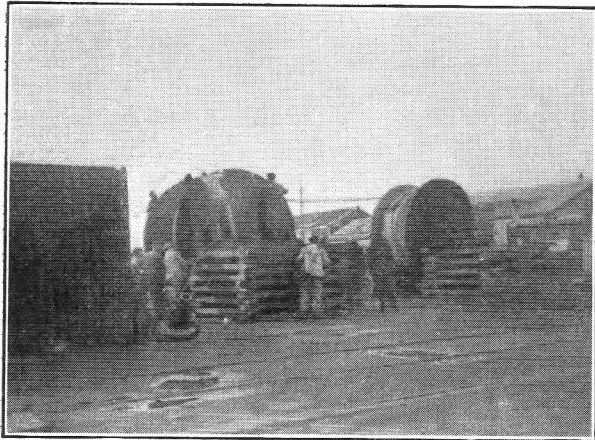
RE-DRUMMING CABLE AT PEMBROKE DOCK.
