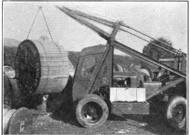
MOBILE CRANE HANDLING HEAVY STORES IN A DEPOT.
