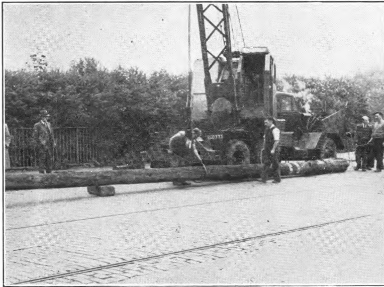
FIG. 3.—READJUSTING THE SLING FOR LIFTING POLE ON TO TRAILER.
