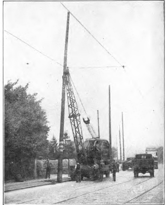
FIG. 1.—POSITIONING THE CRANE.
