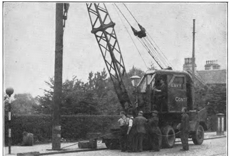
FIG. 2.—LIFTING THE POLE.
