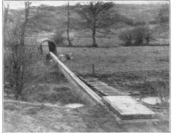
55 FT. (S) POLE AS TEMPORARY SUPPORT FOR STEEL PIPES.
