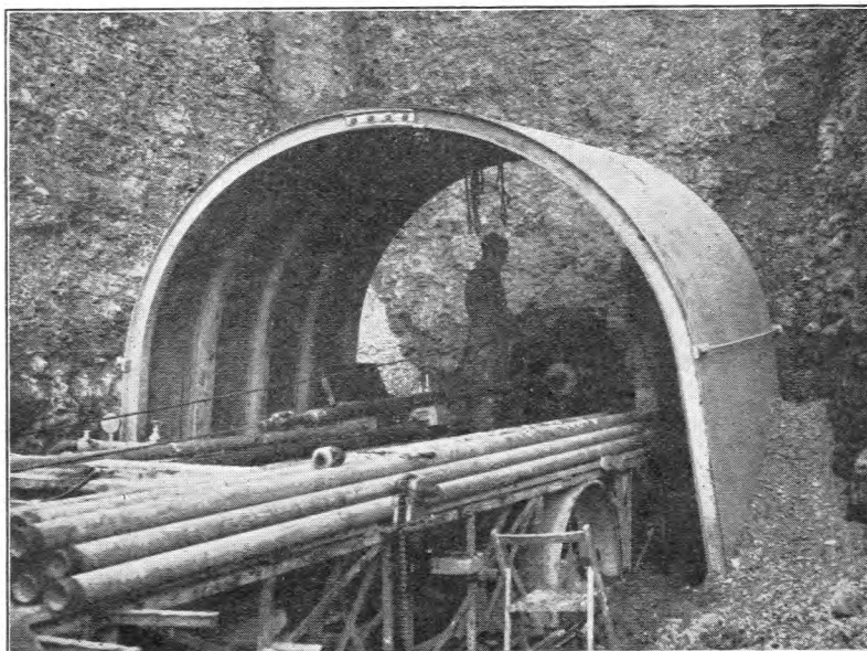
FIG. 8.—DRILLING RIG AT ENTRANCE TO LATERAL BOREHOLE.
