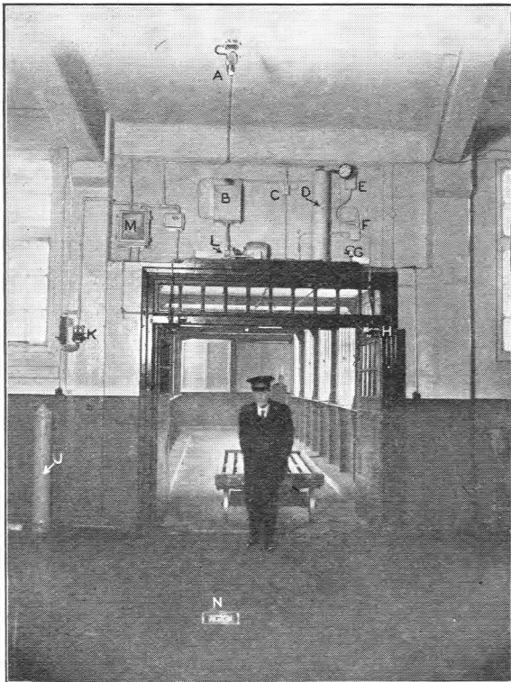
FIG. 3.—HYDRAULIC POWER-OPERATED DOOR.
