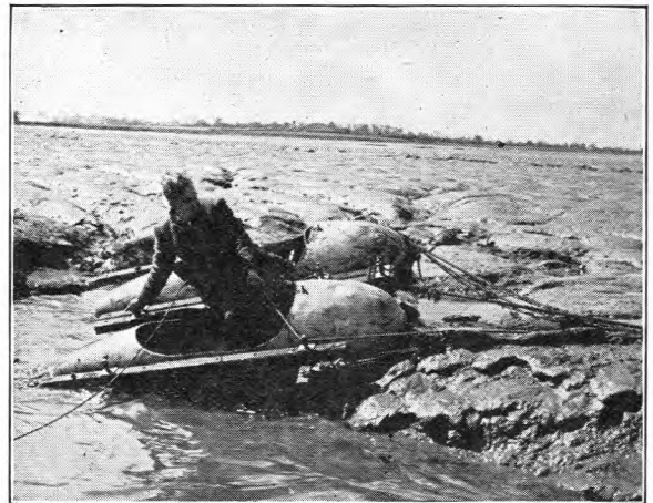
CROSSING A SMALL CREEK. CABLE CAN BE SEEN ENTERING TUBE BELOW DRIVER'S RIGHT ARM.
