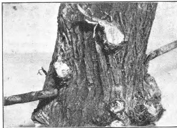
15-PR. PROTECTED CABLE EMBEDDED IN TREE.
