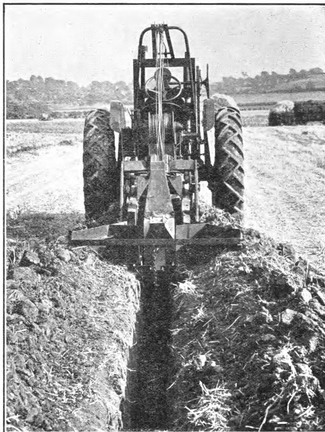
REAR VIEW OF AVELING BARFORD TRENCHING MACHINE TYPE HA2.
