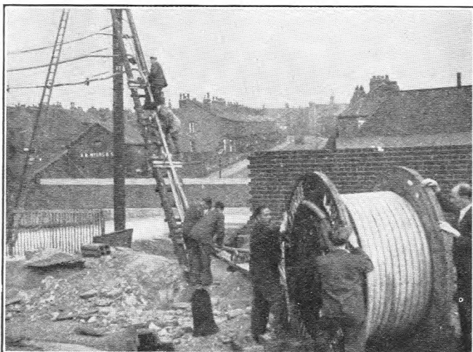
RAMP CONSTRUCTED ON SHEFFIELD SIDE; DRAWING THROUGH OF 3RD CABLE IN PROGRESS.
