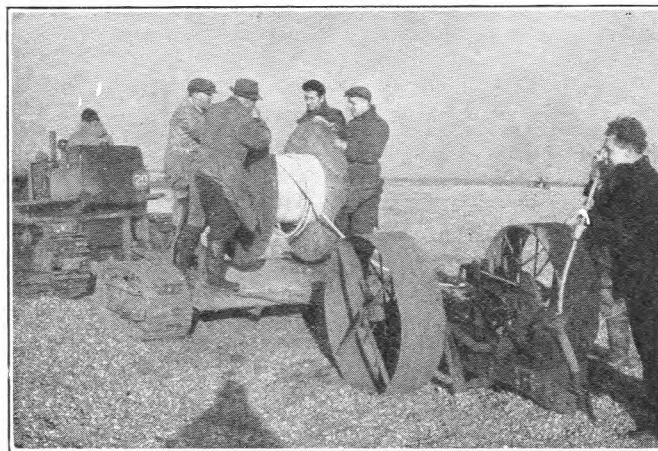
MOLEDRAINING CABLE IN SHINGLE.
