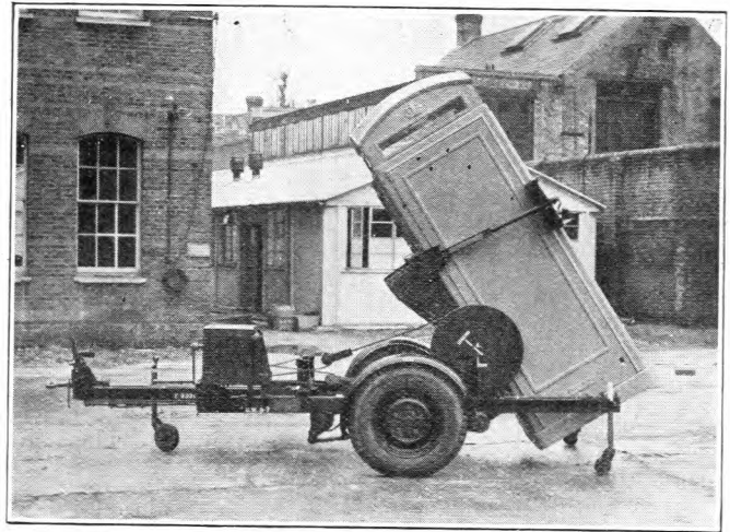
FIG. 2.—KIOSK LIFTED AND BEING TURNED.
