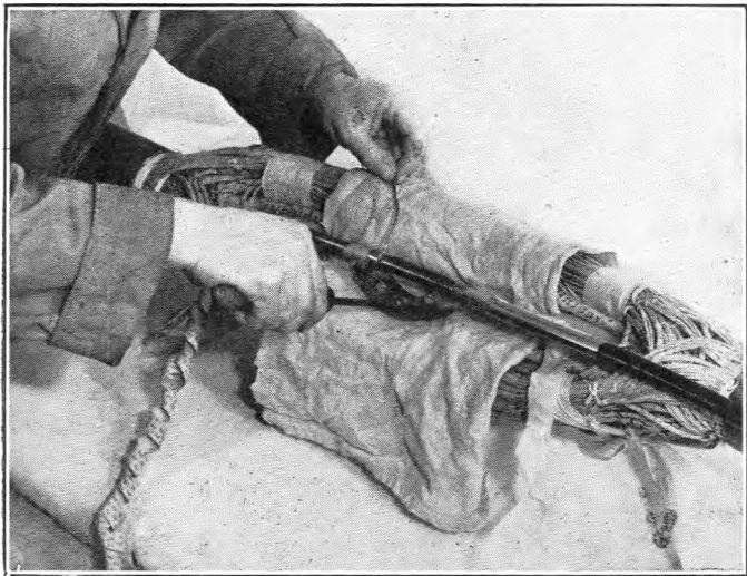
FIG. 8.—NEW JOINT; SOLDERING OPERATIONS ON A COAXIAL PAIR.
