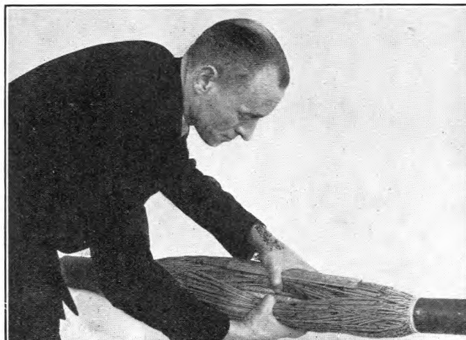
FIG. 2.—BARREL TYPE JOINT COMPLETED; SHOWING LIMITED ACCESS TO COAXIAL PAIRS.
