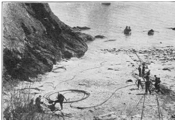
TESTING ONE OF THE SHORE ENDS.
