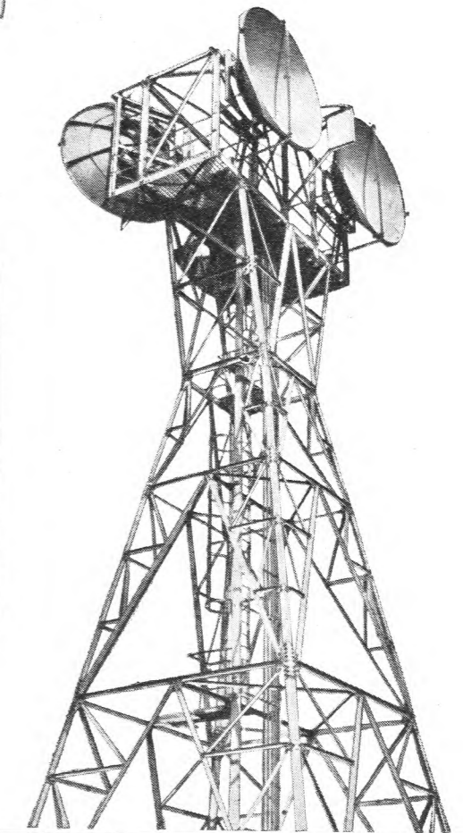
The Microwave Television Link installed between Manchester and Kirk o' Shotts, a distance of approximately 250 miles, employs beamed transmissions over line-of-sight paths. Seven repeaters, the antennæ of one of which is shown above, relay programmes in either direction.
