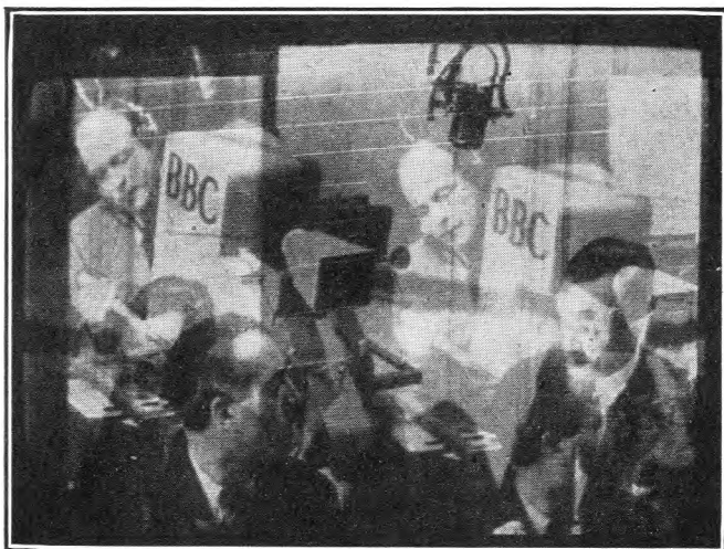
FIG. 5.—PICTURE TRANSMITTED ROUND LOOP LONDON-BIRMINGHAM-LONDON AND SUPERIMPOSED ON ORIGINAL.
