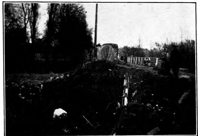
CABLE REPAIRS IN PROGRESS.
