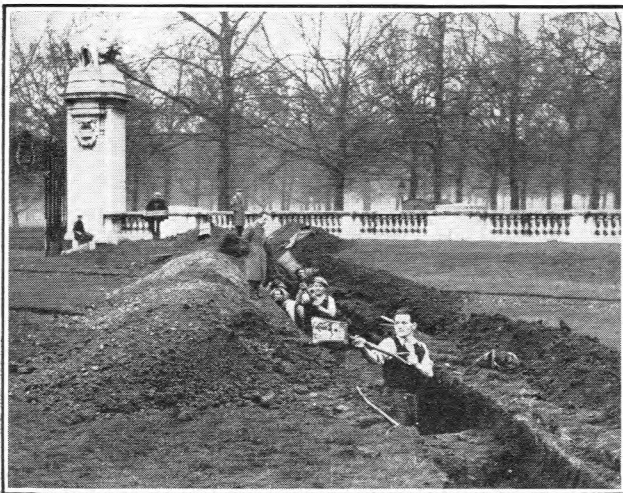
FIG. 2.—EXCAVATING FOR DUCT ROUTE NEAR CANADA GATE.
