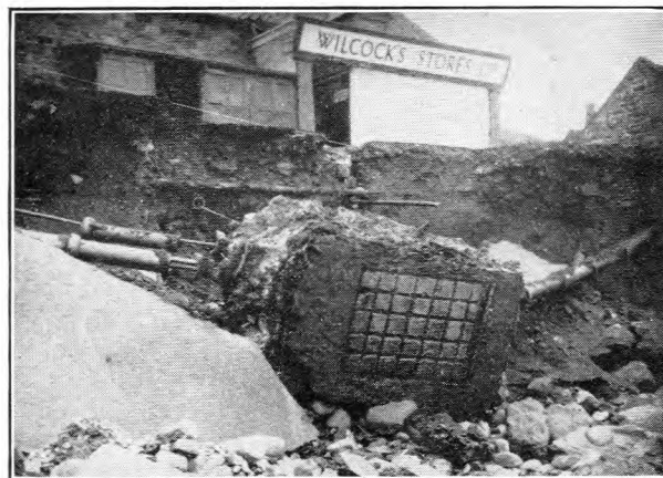
THE JOINT BOX SUSPENDED ON CABLES.
