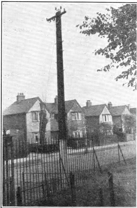
“HALVED” POLE ERECTED.
