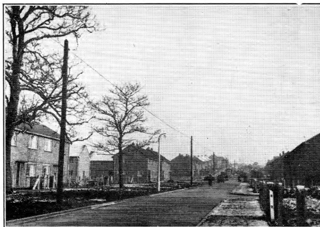
APPEARANCE OF TYPICAL AERIAL CABLE AND DROP-WIRE.
