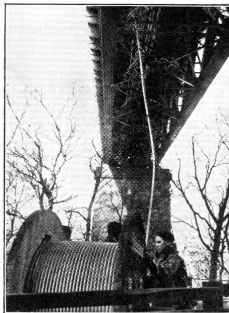
FIG. 6.—CABLING ON THE SOUTHERN APPROACH TO THE BRIDGE.
