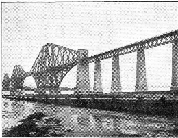
FIG. 1.—GENERAL VIEW OF BRIDGE AND SOUTHERN APPROACH.
