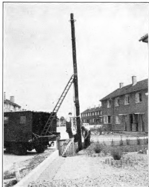
ERECTING A POLE WITH THE DERRICK.
