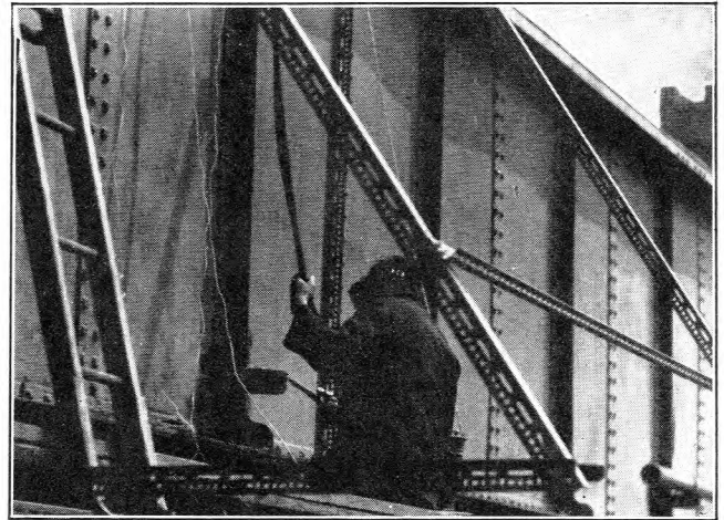
WELDER SUPPORTED BY DEXION FRAMEWORK ATTACHED TO BRIDGE ACROSS RIVER URE.
