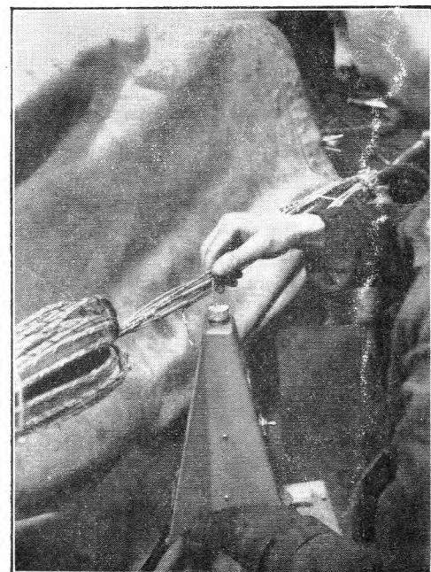
FIG. 9.—SOLDERING ALUMINIUM CONDUCTORS TO COPPER CONDUCTORS.
