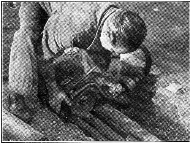
CUTTING THE STEEL PIPE.
