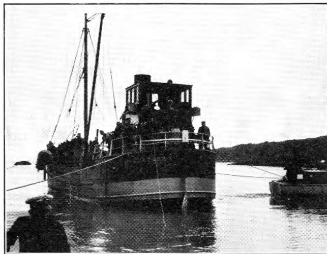
LANDING THE CABLE FROM THE "GLEN ARAY"
