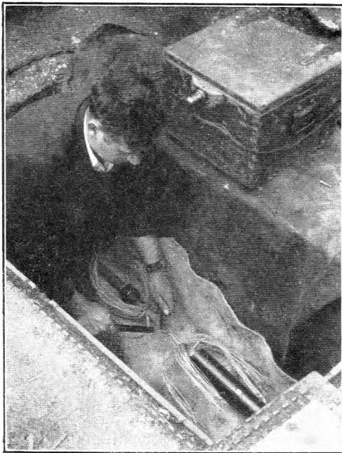
FIG. 6.—WELDING A JOINT IN THE ALUMINIUM CONDUCTORS.
