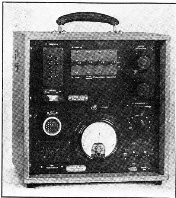
FIG. 3.—BIAS DISTORTION TESTER.
