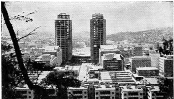
VENEZUELA BIC Construction Co. have undertaken the jointing and supervision of installation of a 448 pair 20 lb trunk cable to improve the telephone service between Caracas and Maquetia. With a route length of approximately seventeen miles, the cable runs wholly in ducts along the side of a newly-constructed auto-road linking the capital town of Caracas with the coast. This contract has been undertaken for the Compania Anonima Nacional Telefonos de Venezuela, the cable being manufactured by BICC.
