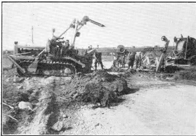
FIG. 11.—ONE OF THE TRENCHING MACHINES AT WORK.
