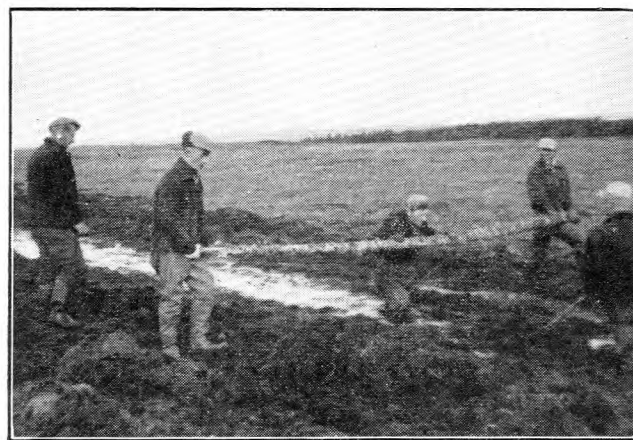
FIG. 14.—TREADING THE CABLE TO THE CORRECT DEPTH.
