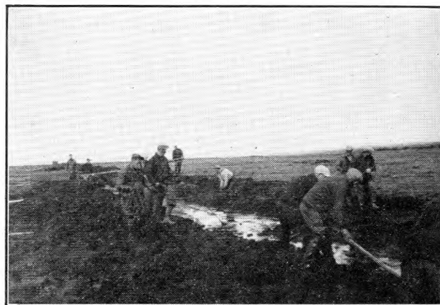
FIG. 13.—WORKING THE CABLE INTO THE TRENCH.
