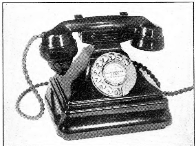
FIG. 7.—COMBINED TELEPHONE AND BELL-SET.
