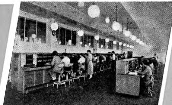
SKYPORT PABX at London Airport, 1956
