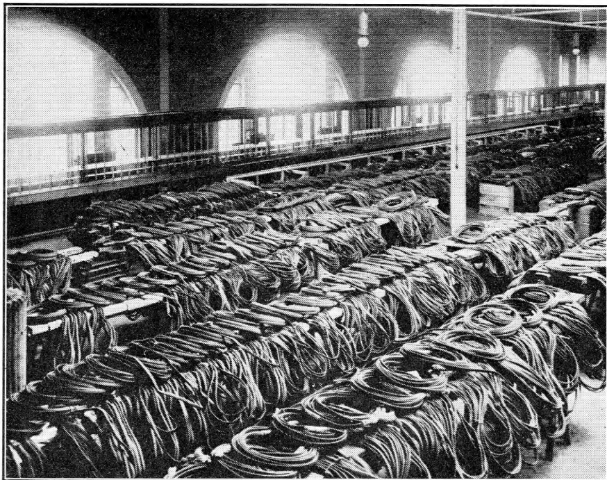
GLASGOW MANUAL TELEPHONE EXCHANGE IN COURSE OF INSTALLATION, 1910.
