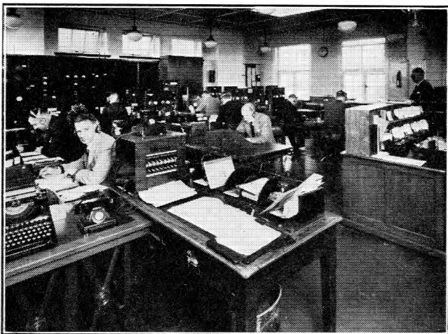
FIG. 3.—RECEIVING ROOM AT BURNHAM RADIO STATION.
