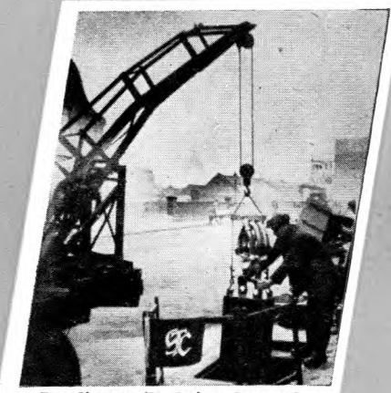
Loading coils being lowered into City street manhole
