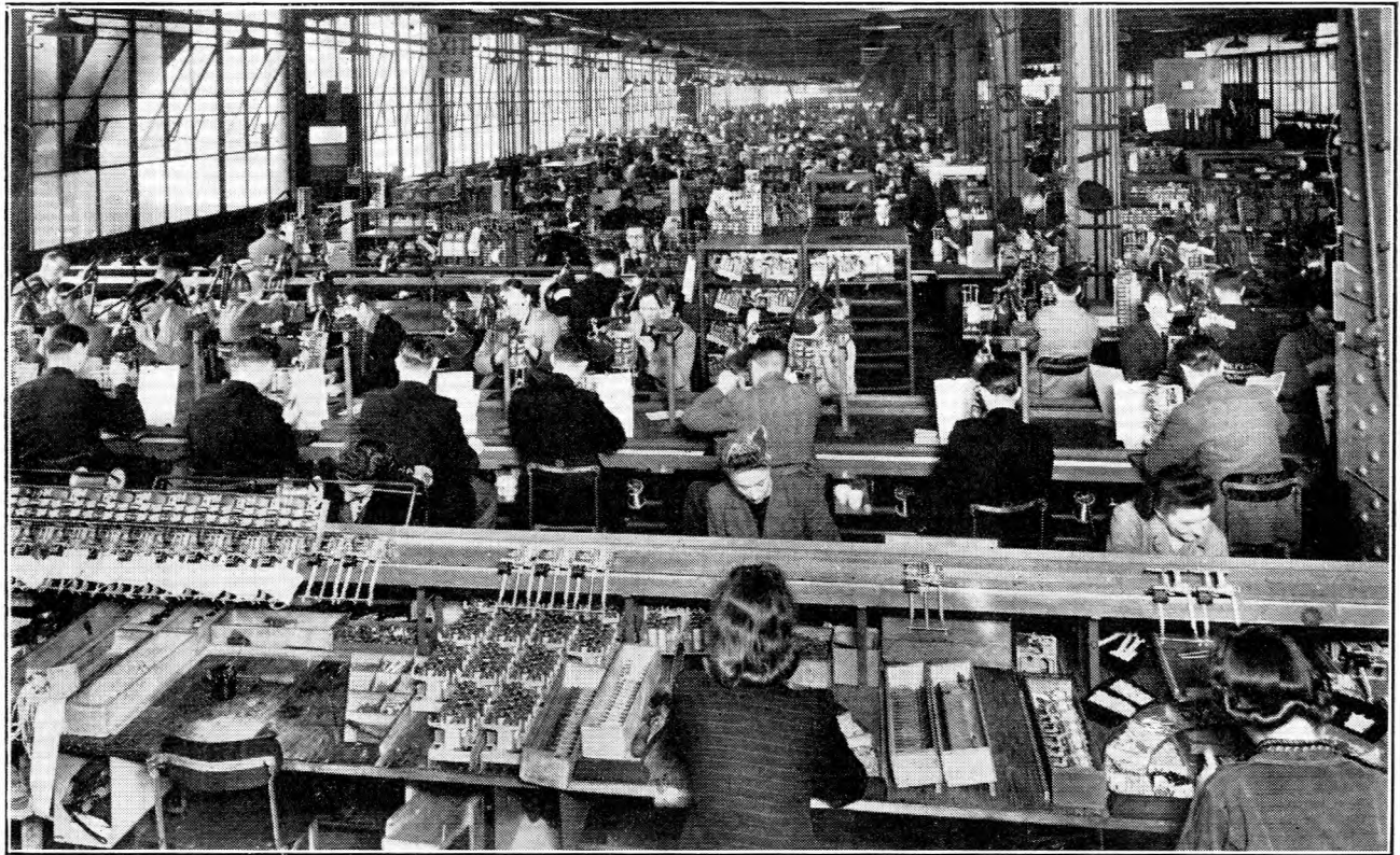
MAIN ASSEMBLY AND WIRING OF 2,000-TYPE SELECTORS.
