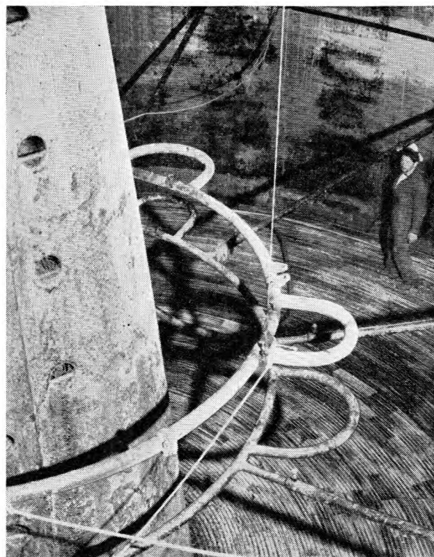
FIG. 7.—INTERIOR OF CABLE TANK, SHOWING CENTRAL CONE, CRINOLINE, AND A "FLAKE" OF CABLE.
