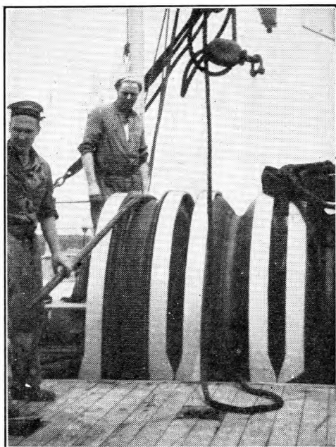
FIG. 2.—BOW SHEAVES, WITH NEW FLAT-TREAD PORT SHEAVE.
