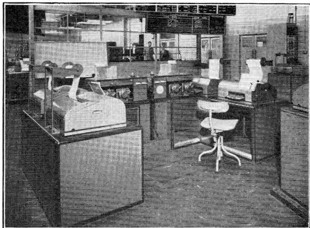
ANOTHER VIEW OF THE RADIO TELE-TYPE MONITORING ROOM SHOWING AUTOMATIC TRANSMITTERS.
