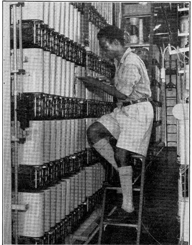
By courtesy of Nigeria Trade Journal and the Federal Information Services LAGOS AUTOMATIC EXCHANGE, EQUIPPED WITH PRE-2,000-TYPE SWITCHES. NEW EXCHANGES ARE BEING EQUIPPED WITH S.E.50 SWITCHES.
