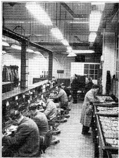
FIG. 9.—ILLUMINATION OF TEST DESKS BY FLUORESCENT LIGHTING.
