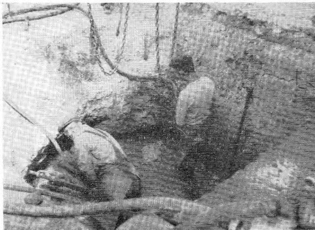
BREAKING UP THE OLD FOUNDATIONS
