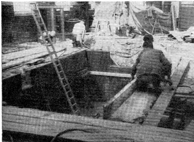
LINING ONE OF THE NEW PITS WITH CORK
